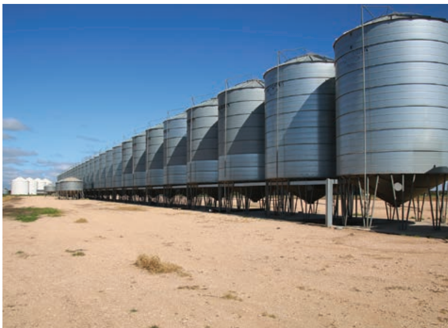
BRETT ROBERTS CAN HOLD APPROXIMATELY 9,000 TONNES OF GRAIN IN VERTICAL STORAGE, WITH ADDITIONAL CAPACITY IN SHEDS, FIELD BINS AND GRAIN BAGS, WHICH IMPROVES HARVEST EFFICIENCY AND MARKETING FLEXIBILITY.
