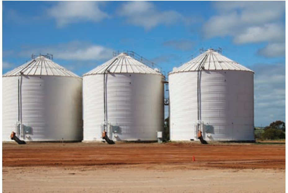
BRETT’S VERTICAL UPRIGHT SILOS ARE SEALED AND FITTED WITH FANS AND OTHER MECHANISMS TO MANAGE MOISTURE AND TEMPERATURE LEVELS OF GRAIN IN THE STORAGES.
